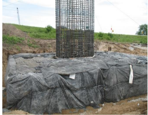
(b) Footing covered with insulation blanket
